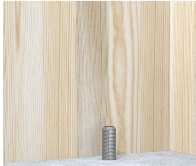
Figure 1 Place the tie-down anchor in concrete or bolt in timber or steel
